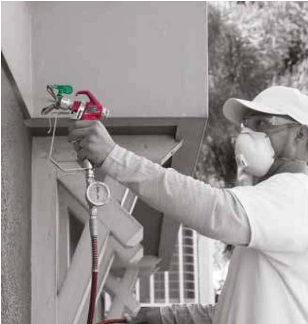
Latex emulsion paint through a standard 517 tip at 70 bar
